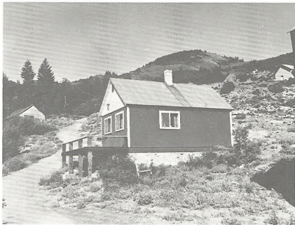
FIGURE 2-39. This house is a prefabricated structure placed on a mortared rubble foundation of undetermined date. It has no historic architecture qualities and was placed on the foundation in 1970 (Block 1, Lot 25½).
